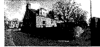
Existing view from South West
