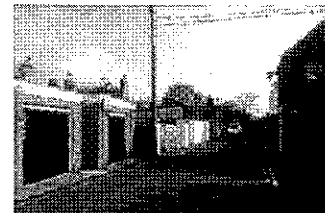
Albyn Terrace Lane – Liner edge of lane broken up by large contemporary openings and garages.
